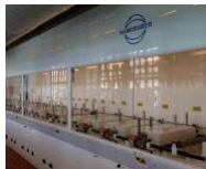
Ramgraber automatic plating line
